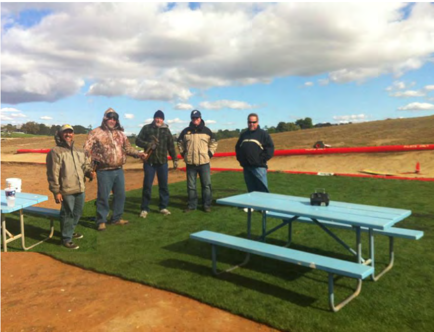
New artificial turf installed at the Torrey Pines Gliderport picnic table/pit area by L-R: Ray, Kevin, Mike, Sean, Robert (Ray P. & Kevin B.)
