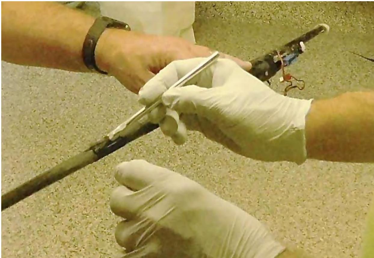
Next, we removed the excess epoxy from the joint by blotting with paper towels and then toilet paper. It's hard to make this too dry; you want to remove just about as much as you can reasonably do. During the process, we're checking the tow position and pushing things around as needed to get a good distribution of carbon fibers around the joint.
