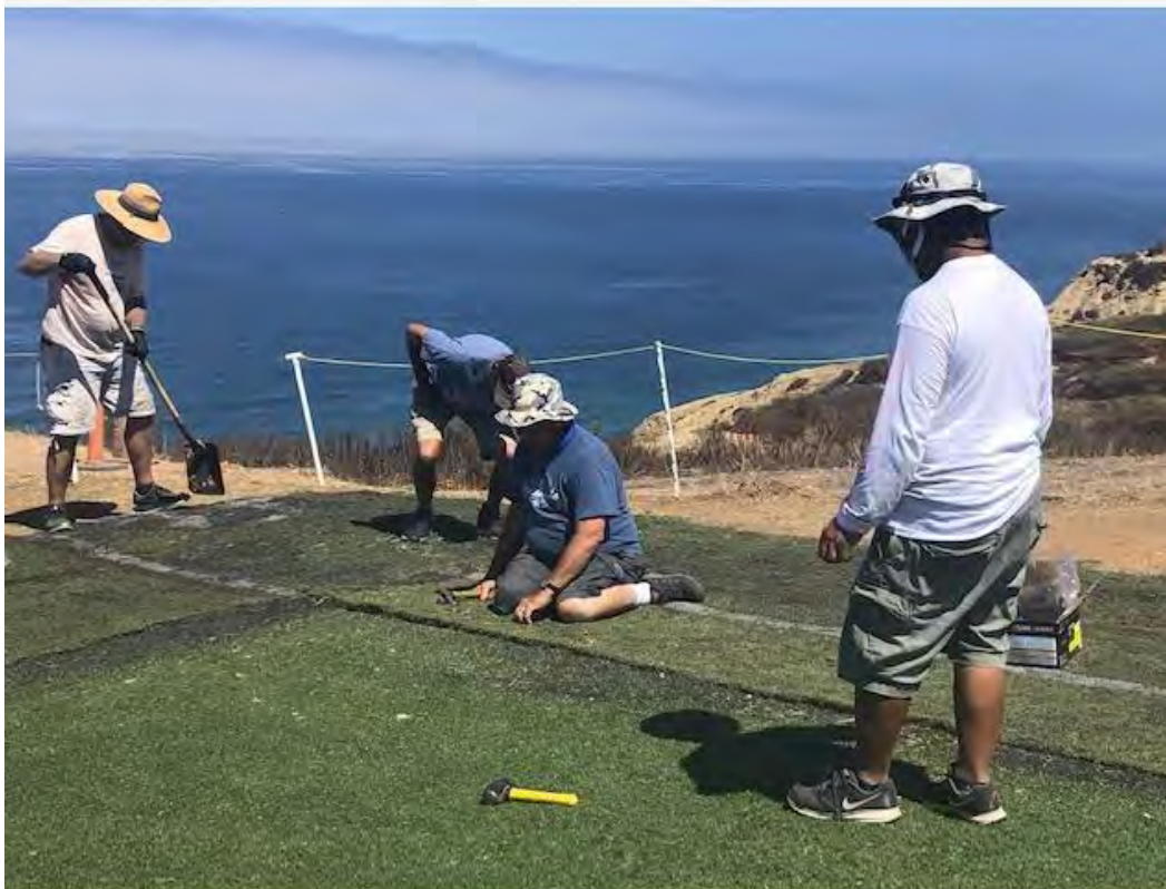
From L to R. Thomas Moller, Mark Anderson, Craig Hansen, and Ray Pili. We used long nails to fasten the turf onto the dirt. (Mark Baldacchino photo)
