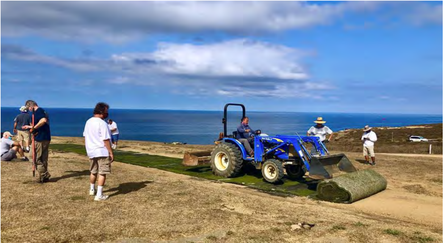
Unrolling with the infill still in the AstroTurf. Four more rolls are going here to double the width. (Mark Baldacchino photo)
